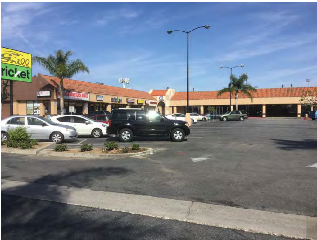
View of subject property to the northwest. 16257-16255 San Fernando Mission Blvd., Granada Hills, 91344
