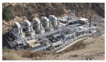
Sunshine Canyon Landfill is home to a new landfill gas-to-energy (LFGTE) project. The 20-megawatt renewable energy project is capable of generating enough electricity to power nearly 25,000 area homes.
